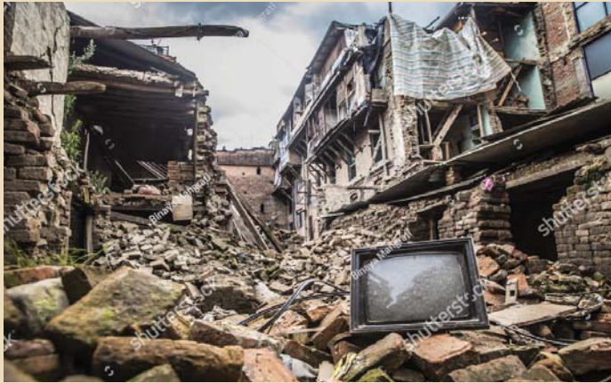
Gambar 2. Kerusakan Akibat Gempa Bumi (sumber: https://www.shutterstock.com/image-photo )
